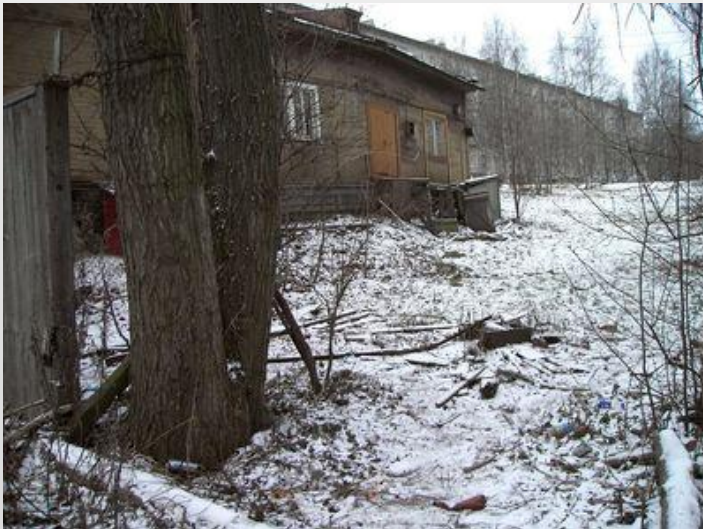
The dangerous communicating courtyard
